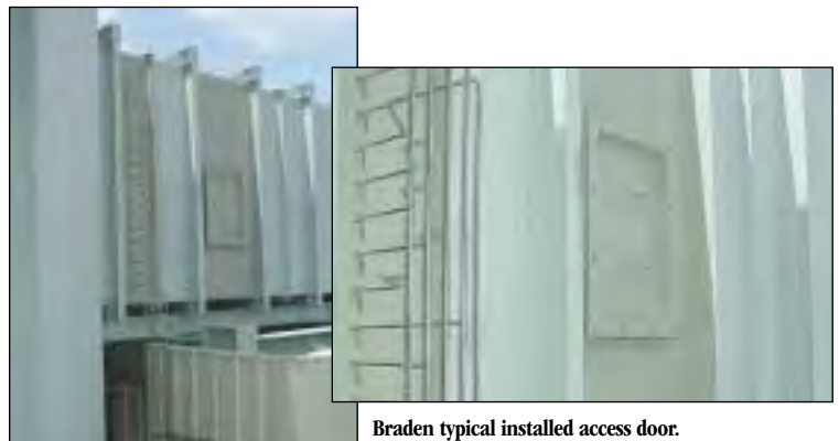
Braden Fogging System located at a Texas gulf coast chemical company sized for a frame 7EA gas turbine.
