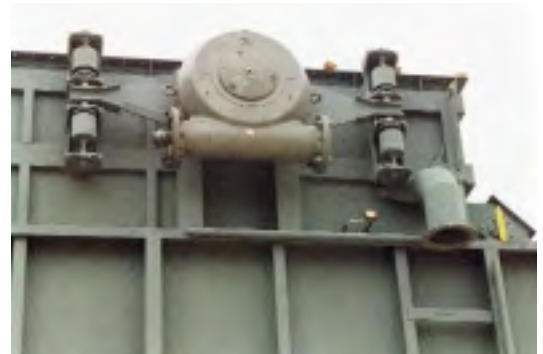
Electric actuator for a toggle linkage drive, spring mounted for temperature compensation. Electric drive systems use an actuator to drive a self-locking gearbox.
