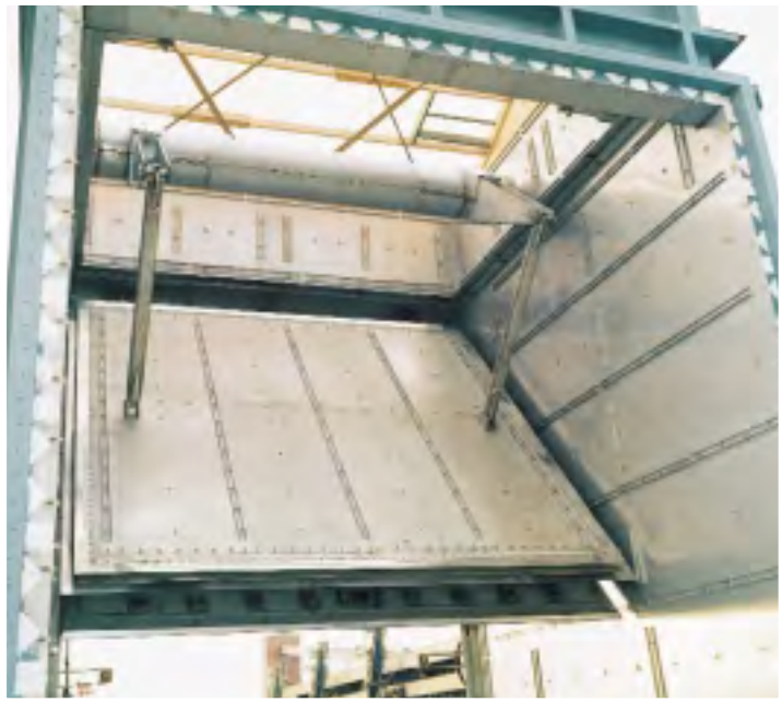
Toggle linkage mechanism installed on a FS-9E diverter damper.
