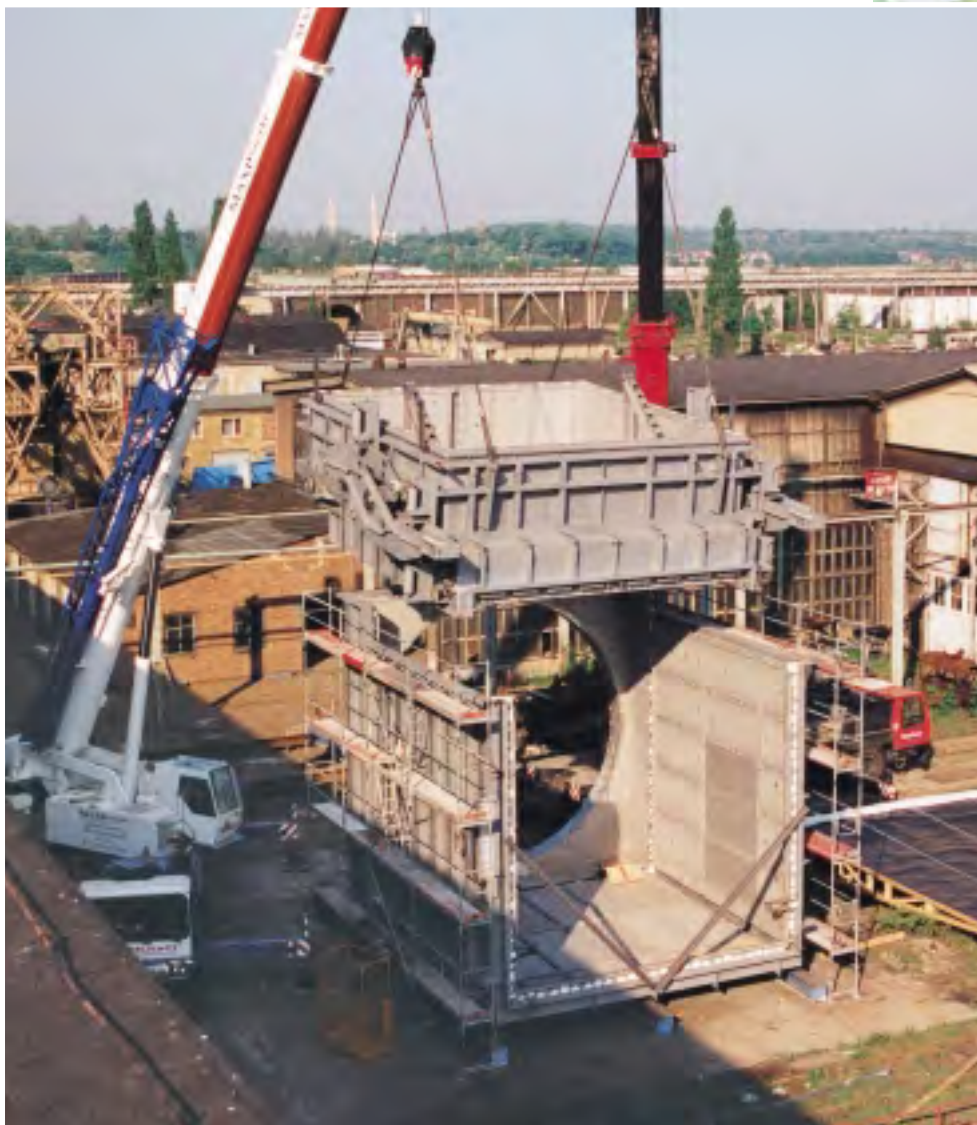
Shop pre-assembly of V94.3A diverter for functional testing.
