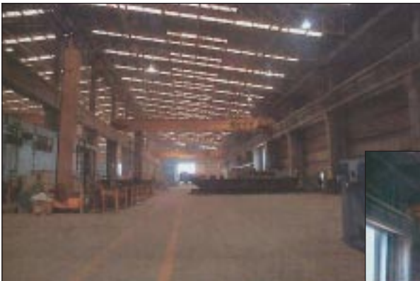
The interior of Braden's manufacturing facilities in Monterrey, Mexico.
