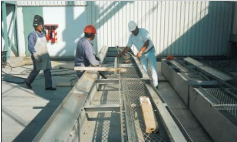
Braden Construction: evaporative cooler installation, Siemens V94.2, South America
