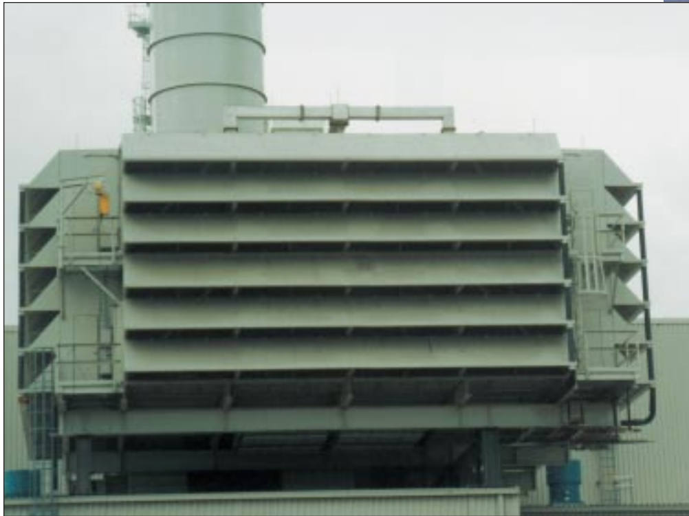
Barrier filter with anti-icing for Siemens V94.3A in Argentina, SA.
