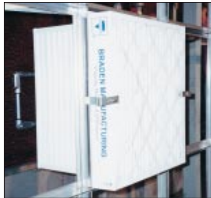
Two-stage Barrier Filter House
