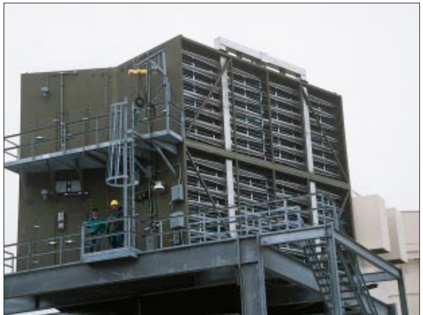
Barrier filter with cooling coils and an anti-icing system for an ABB 11N1 in Nebraska, USA.
