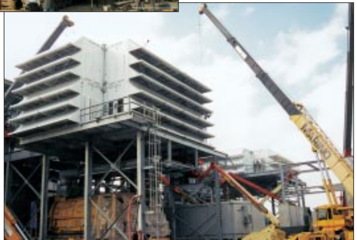
Siemens V84.3A Barrier Filter with Anti-Icing System in Connecticut, USA.
