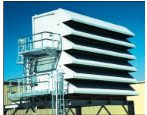
Barrier filter for a GE frame 6B in Thailand.
