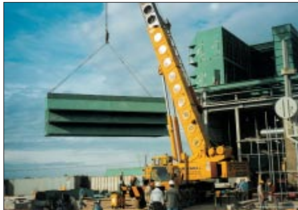
Siemens V84.3A Barrier Filter with Anti-Icing System in Connecticut, USA.
